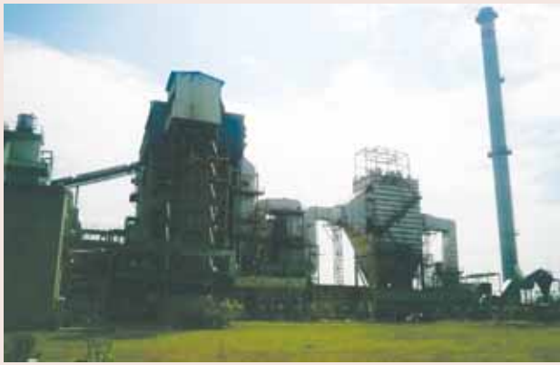
Boiler: Capacity 120 TPH, 87 ata, 510°C
