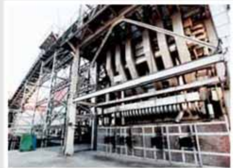
National award winning sugar plant Shri Swami Samarth S.S.K., Solapur, Maharashtra powered by Uttam boiler
