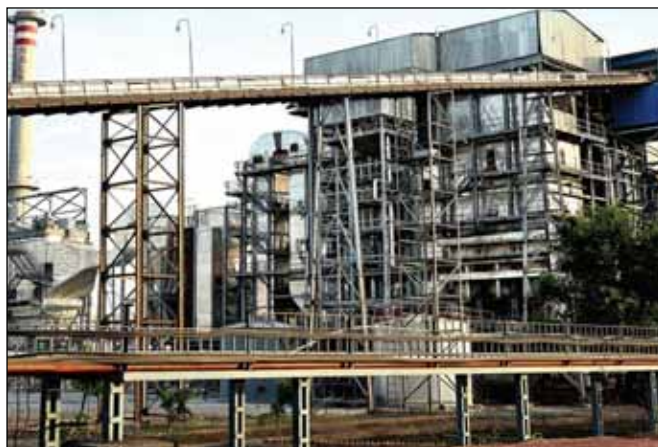
M/s NSL KSL (P) Limited (25 TPH, 65 kg/cm 2 , 485°C boiler)
