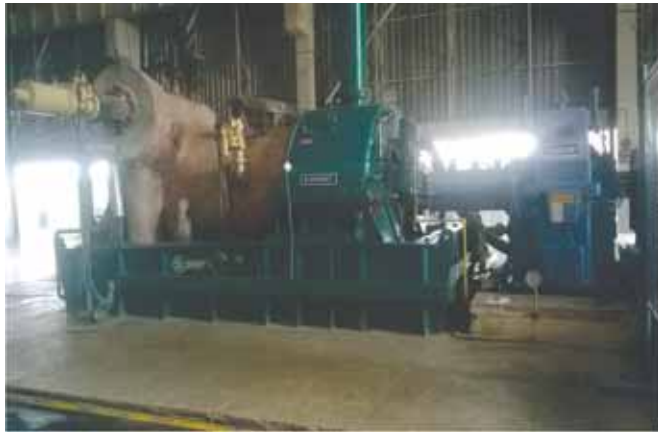
Turbine: Extraction cum condensing; Capacity 22 MW, 87 ata
