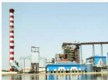
12.5 MW co-generation & EPC for Shivratna Udyog, Solapur, Maharashtra with 70 TPH bagasse fired Uttam boilers
