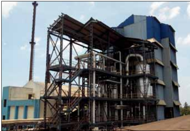
Biomethanated Spent Wash Evaporation
