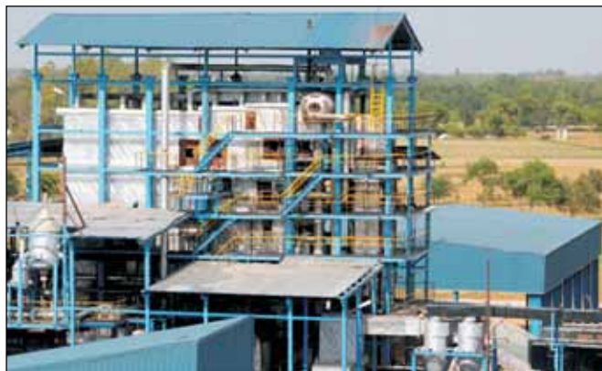
M/s Wave Distillery (25 TPH, 45 kg/cm 2 , 440°C Boiler)
