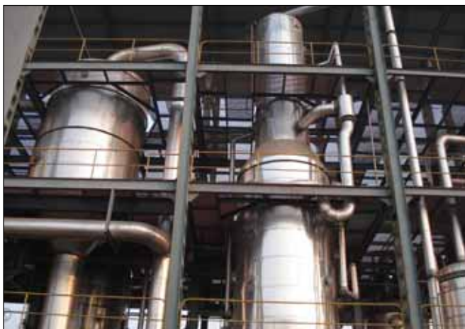
Vinasse Evaporation System
